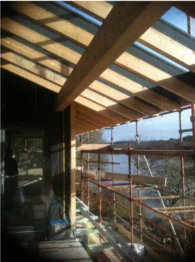
30.11.2010 Patent Glazing fitted
