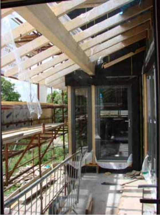
26.08.2010 – Windows in getting ready for air testing
