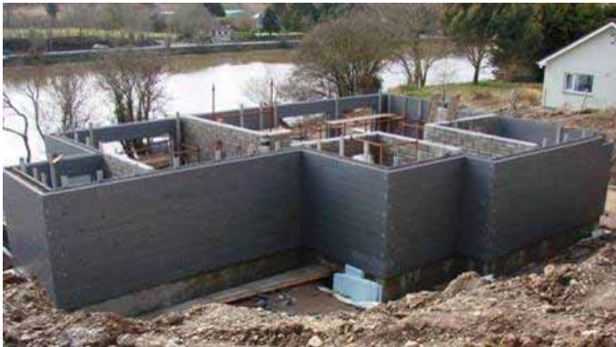
24.03.2010 – Cross walls in, independent and without cold bridging
