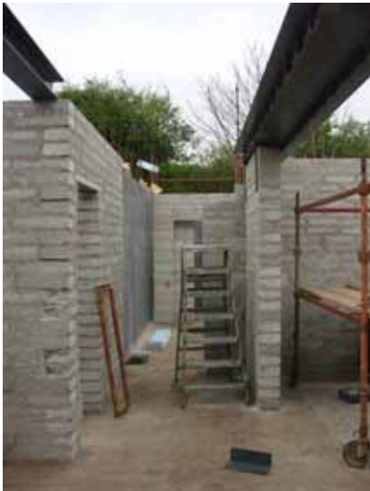
05.05.2010 – getting ready for 1 st floor
