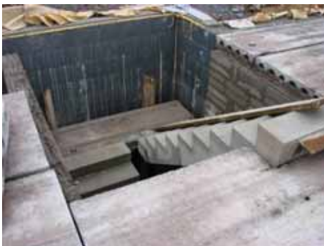
19.05.2010 – slabs on and pc stairs in – again no cold bridging
