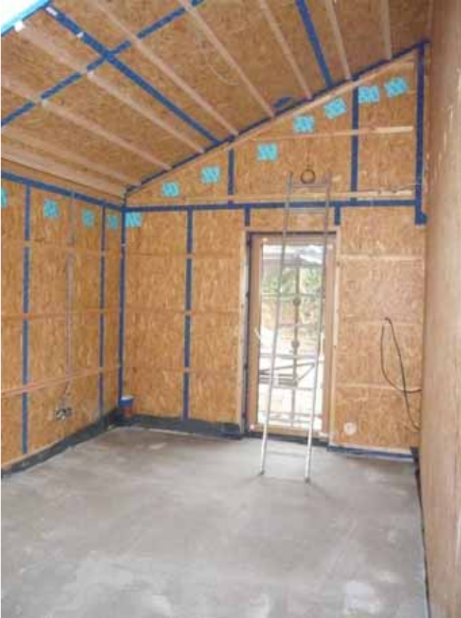
26.10.2010 Cellulose Insulation pumped in walls ready for Airtight testing
