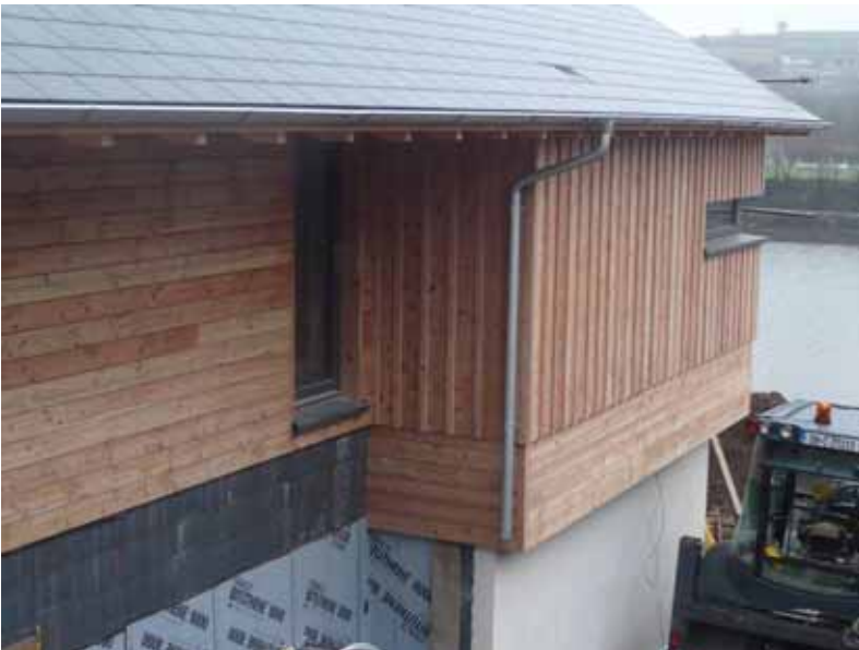
16.12.2010 External Cladding really taking shape, lower walls ready from Pelicolour cladding
