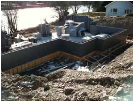
09.03.2010 – ICF well underway
