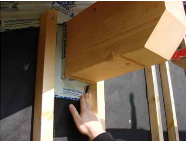
13.10.2010 External Membranes, taped and sealed
