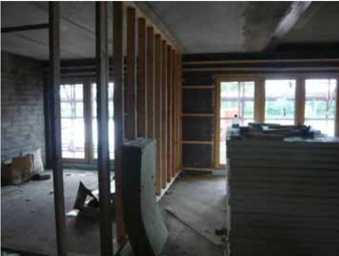
13.09.2010 First fix studwork underway on ground floor – ahead of screed
