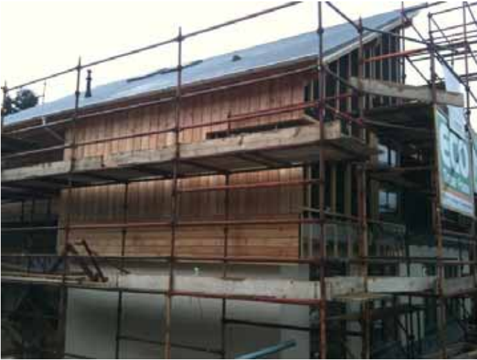
30.11.2010 Larch cladding started on West elevation
